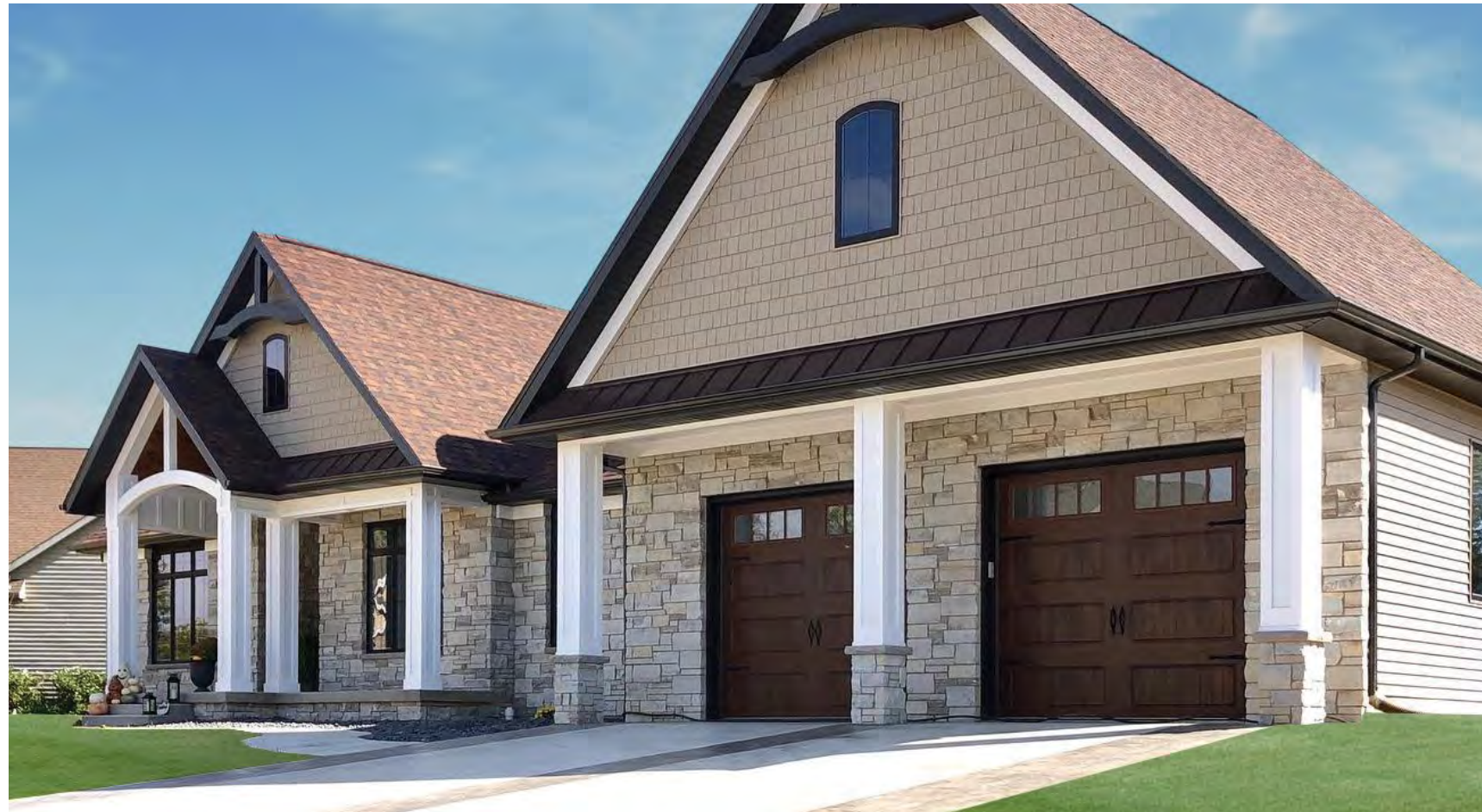
BELOW: Mountain Ridge Dimensional | PROJECT BY: Illinois Brick Company
