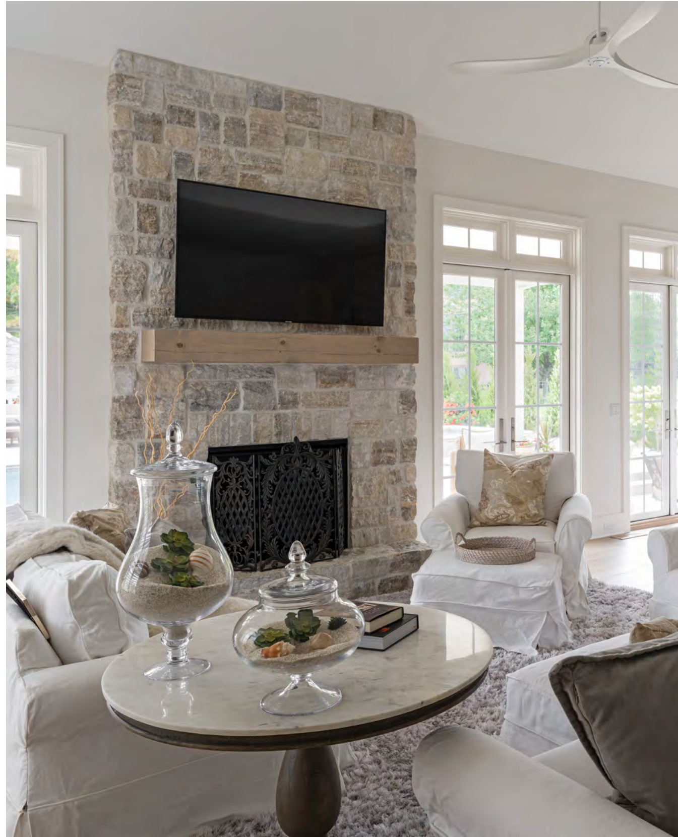
NOTE: The stone in this photo has been grouted with white mortar and the joints are not raked to create a unique look.
